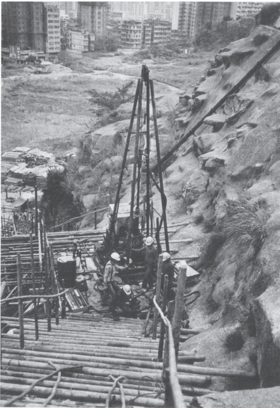
Figure 12. Bamboo scaffolding used to support drillrigs on Hong Kong slopes
